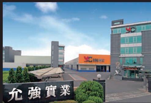
總公司 Headquarter 溪州廠 Shijou Mill (≅ 47,000m 2 )
